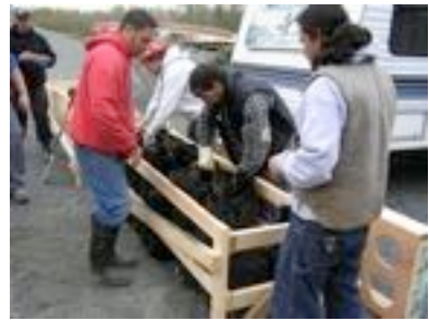
6) Remove Top Frame, seal Bags with cable/rebar ties
