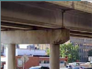
FIGURE 2 MN I35 BRIDGE PIER DAMAGE (2012)
