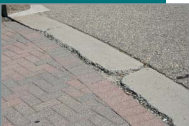
FIGURE 3 BURNSVILLE, MN BUS TERMINAL, CONCRETE DEGRADATION (2012)
