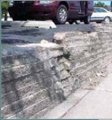
FIGURE 1 EFFECTS OF DRAINAGE AND SALT EXPOSURE FROM PARKING LOT ABOVE SRW (REF. 6., FIGURE 14)
